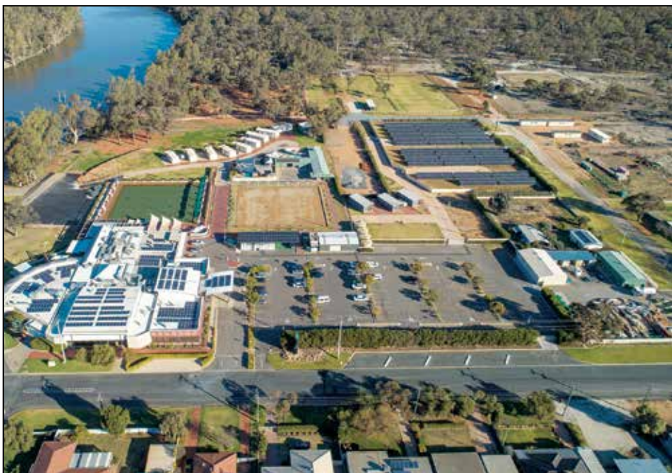
Aerial view of the magnificent Euston Club Resort and the solar Microgrid.
